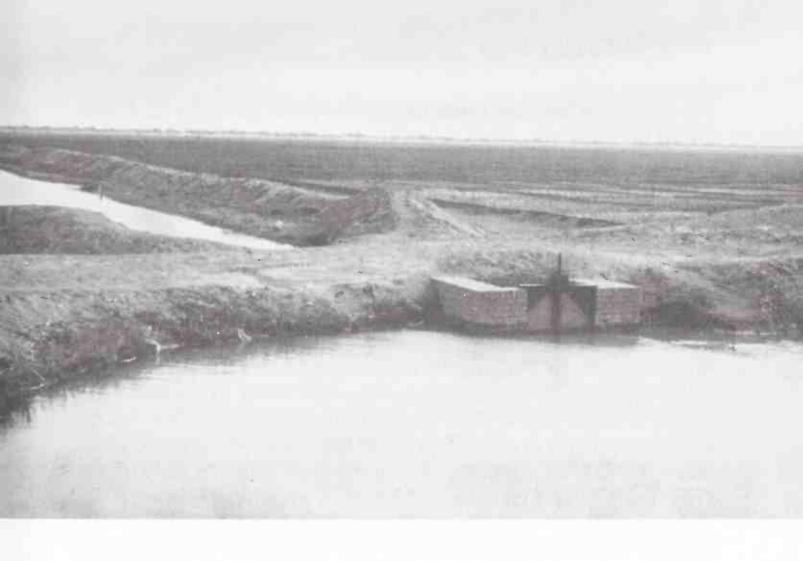
Control device for switching water flow to one of the many canals used for irrigation in Al Jazirah, south of Khartoum Courtesy Embassy of the Republic of Sudan, Washington
